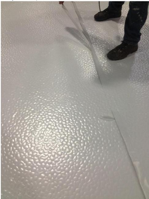
5. After the roof is on the interior tape tab should be smoothed out and adhered to the adjoining panel.
